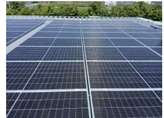
Approximately 1,000 solar panels installed on the roof of the warehouse building
