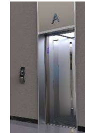
Left: Elevator boarding area equipped with the destination registration system DF-f
