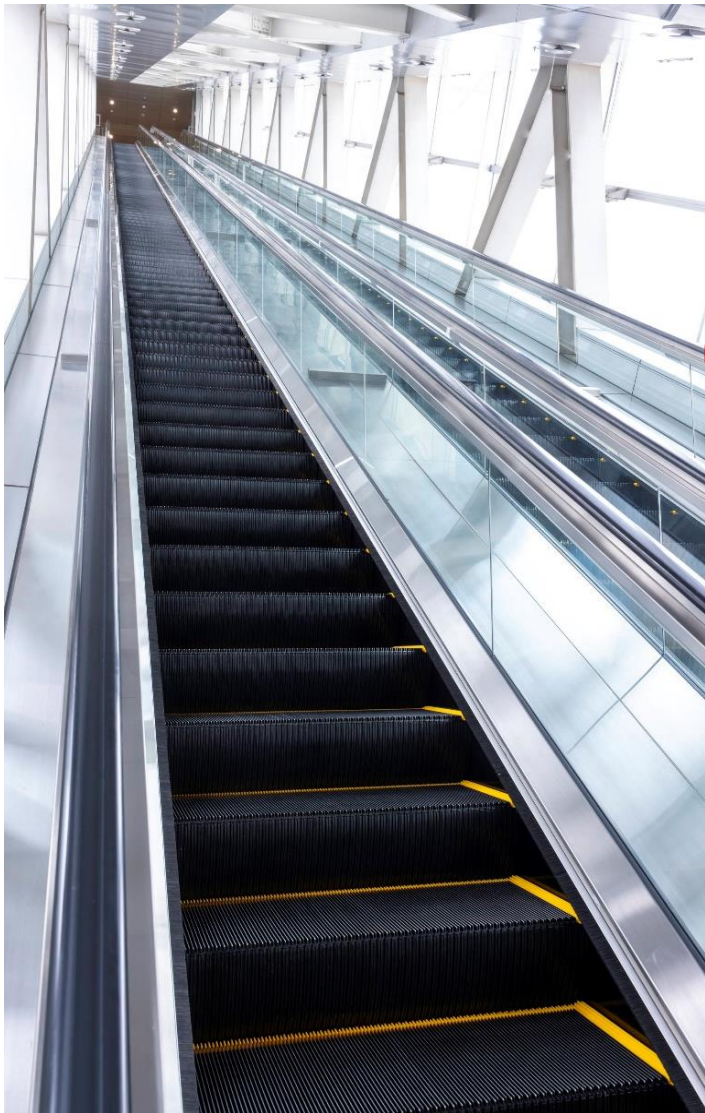
Longest Fujitec escalator in Japan (after renewal)
