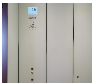
Elevators are button-less, as destination floors are automatically registered
