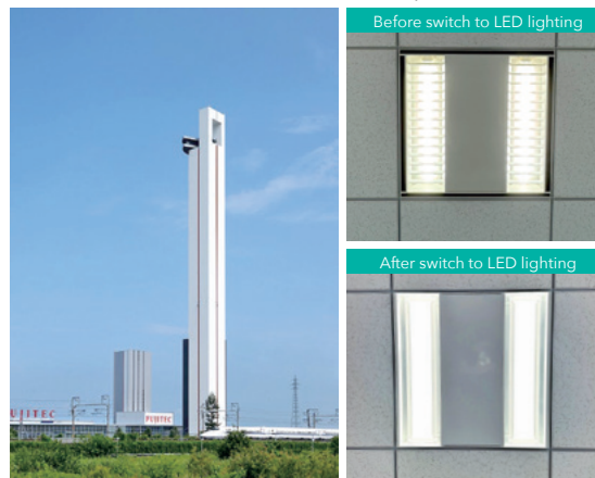
Lighting fixtures in the research wing at Big Wing headquarters have been fully converted to LED.
