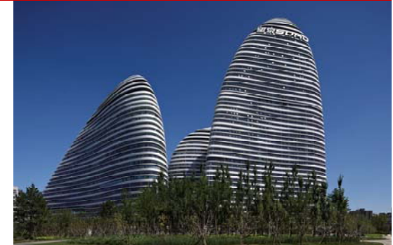
Wangjing SOHO (China)
