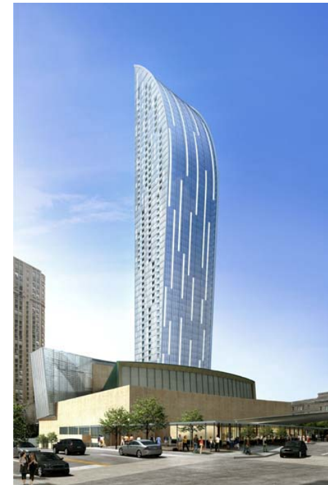
The L Tower (Toronto, Canada)
