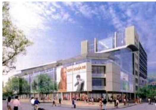
Fujitec Singapore A large commercial facility 'City Square Mall'
