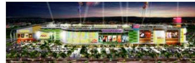
Fujitec Malaysia A large commercial complex 'Jaya Jusco Bukit Tinggi'
