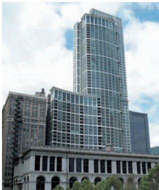
Heritage at Millennium Park
