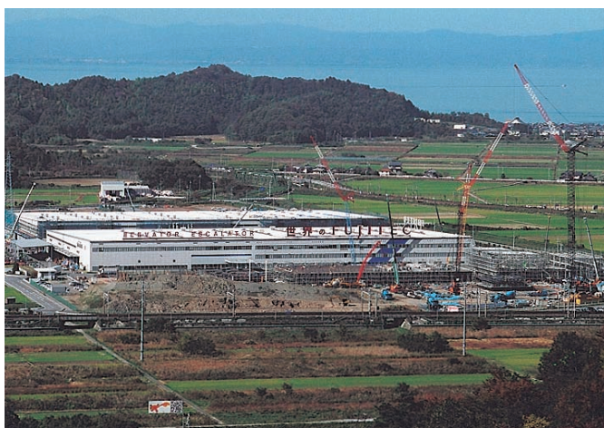
Progress of construction
