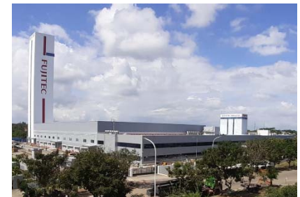
India Plant and Research Tower (Chennai, India)
