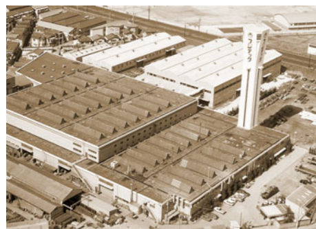
Osaka Plant featuring a 53-meter high elevator research tower (1965)
