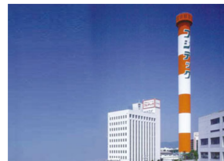
World's tallest and largest elevator research tower at that time (1975)
