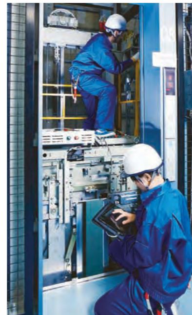
Elevator maintenance operations
