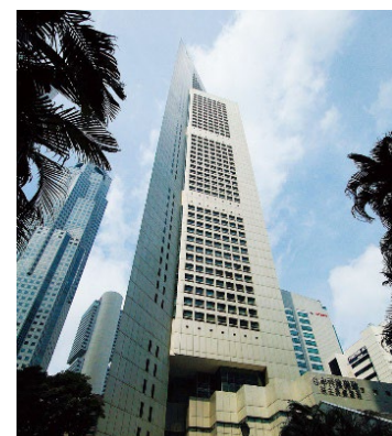
One Raffles Place undergoing modernization work
