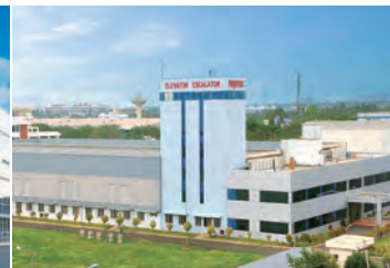
FUJITEC INDIA PRIVATE LTD.
