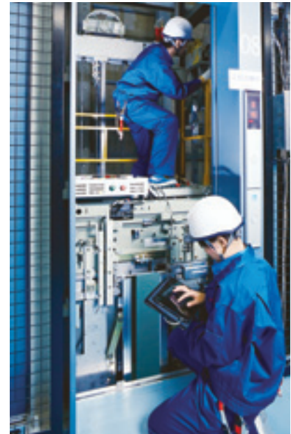
Elevator maintenance operations
