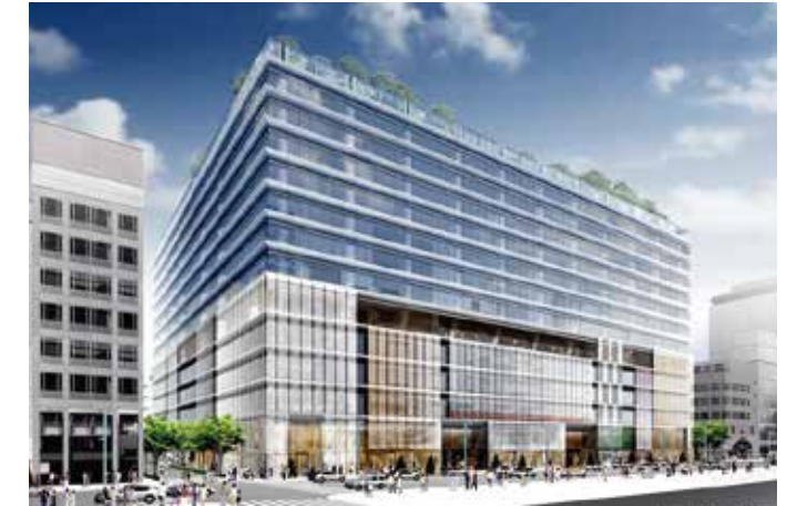
Ginza 6-Chome District 10 Category 1 Urban Redevelopment Project (tentative name) (Tokyo) This redevelopment project involves integrating two districts that include the vacant site of the former Matsuzakaya Ginza store in Ginza, Chuo-ku, with the aim of establishing an international retail, business and tourism base. Fujitec received orders for a total of 76 elevators and escalators for a large-scale multi-purpose building.
