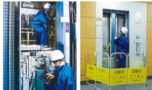
Elevator maintenance operations
