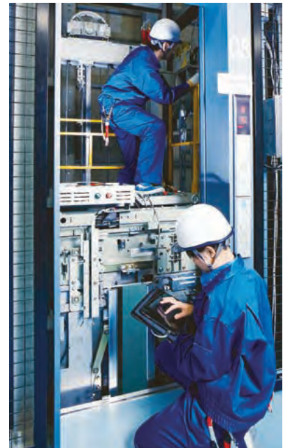
Elevator maintenance operations
