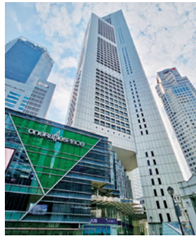
OUB Centre (Singapore) Modernization/Completed The building constructed as the tallest building in Asia in 1986. There are 19 elevators installed.
