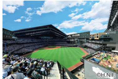
ES CON FIELD HOKKAIDO New Installation/Completed The Japan's first natural-turf stadium with a retractable roof. There are 13 elevators and 14 escalators installed.
