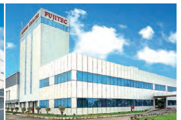
FUJITEC INDIA PRIVATE LTD.
