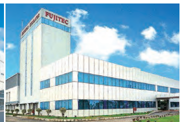
FUJITEC INDIA PRIVATE LTD.
